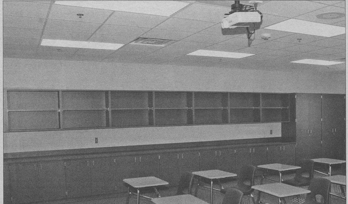
Every classroom features a multimedia projector and smartboard as well as ample storage.
